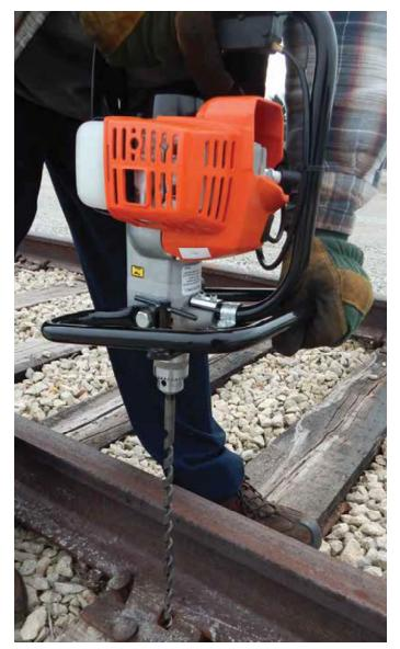
The Racine Gas Tie Drill is designed to pre-drill holes in wood ties for lag screws, bridge timber screws, and crossing projects.
